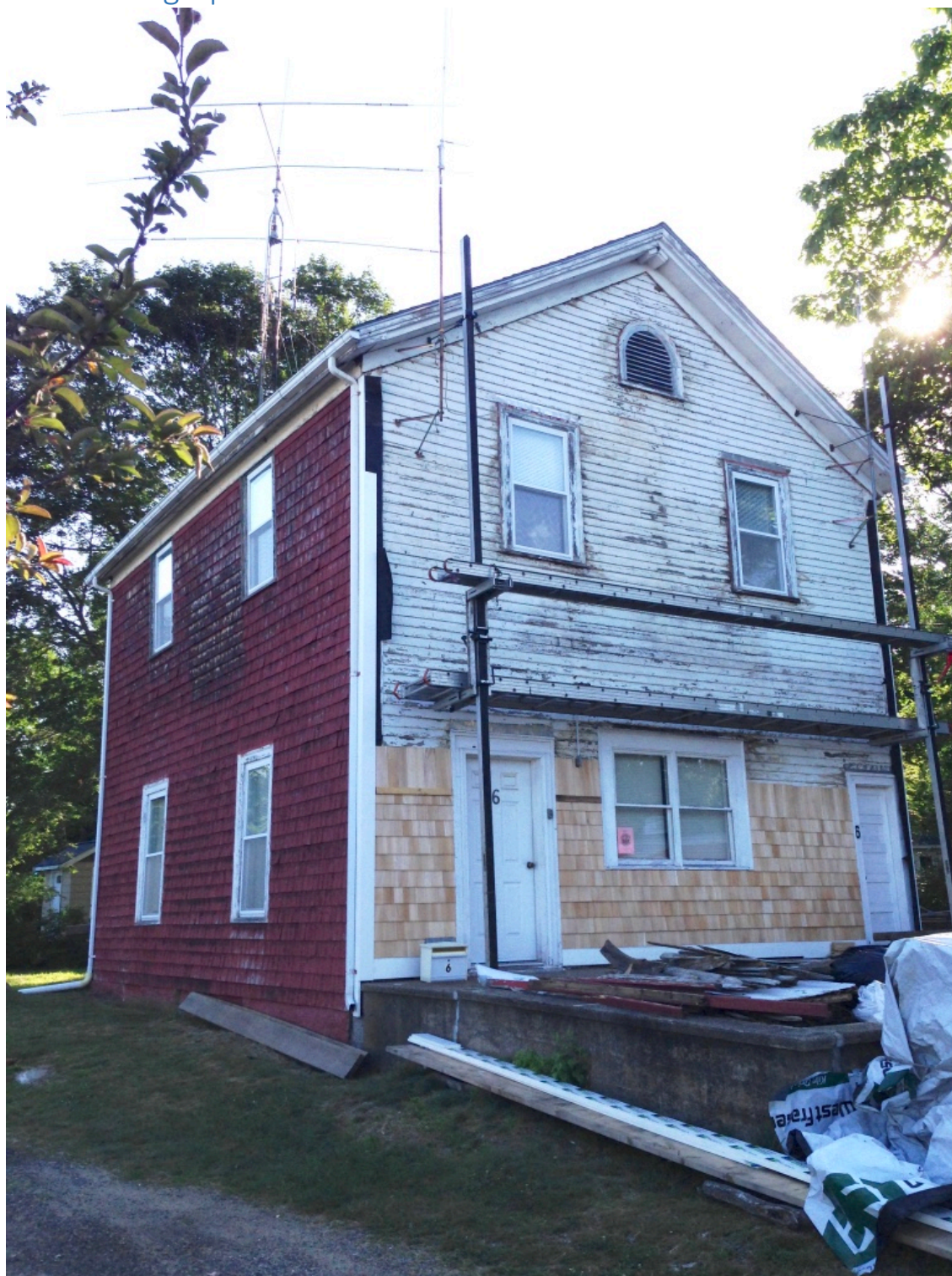
Figure 1. Exterior of the building during re-shingling, 2015. Original shingles were installed over the clapboards in 1980 and painted. New shingles were applied over the clapboards to allow air circulation behind the singles for longer life.
