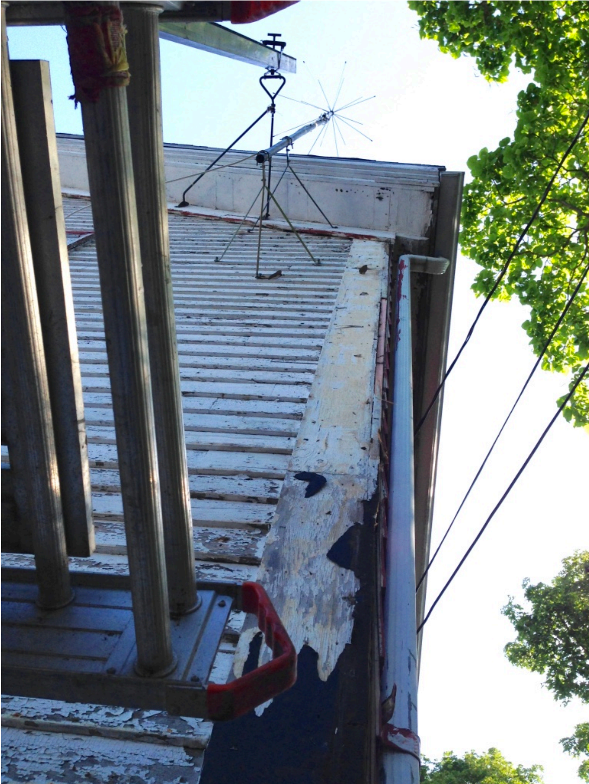
Figure 3. View of right front corner with shingles stripped
