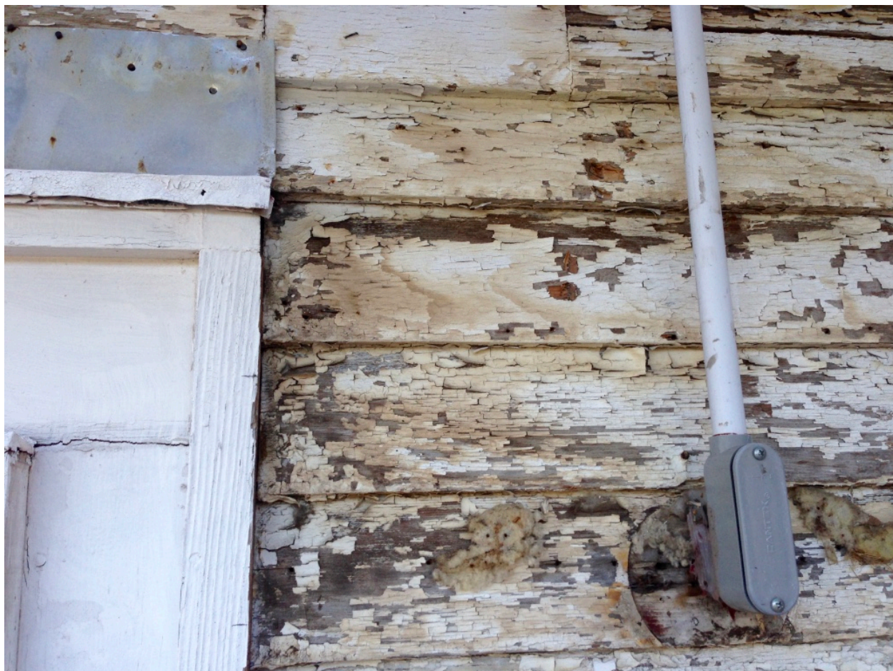
Figure 2. Detail of clapboard condition near the front door. Cedar shingles were applied over the clapboards in 1980.
