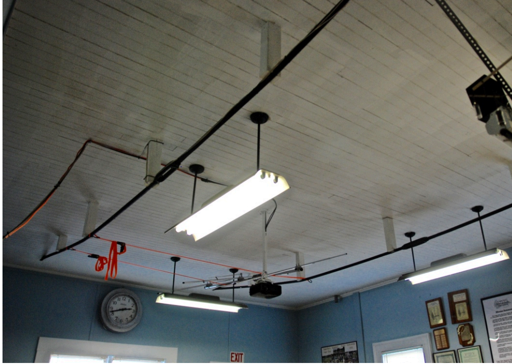
Figure 4. Second floor iron rod suspension support. Rods probably support floor at previous column locations of the original school house. Support system gives unobstructed space across the 20.5' width of the room.
